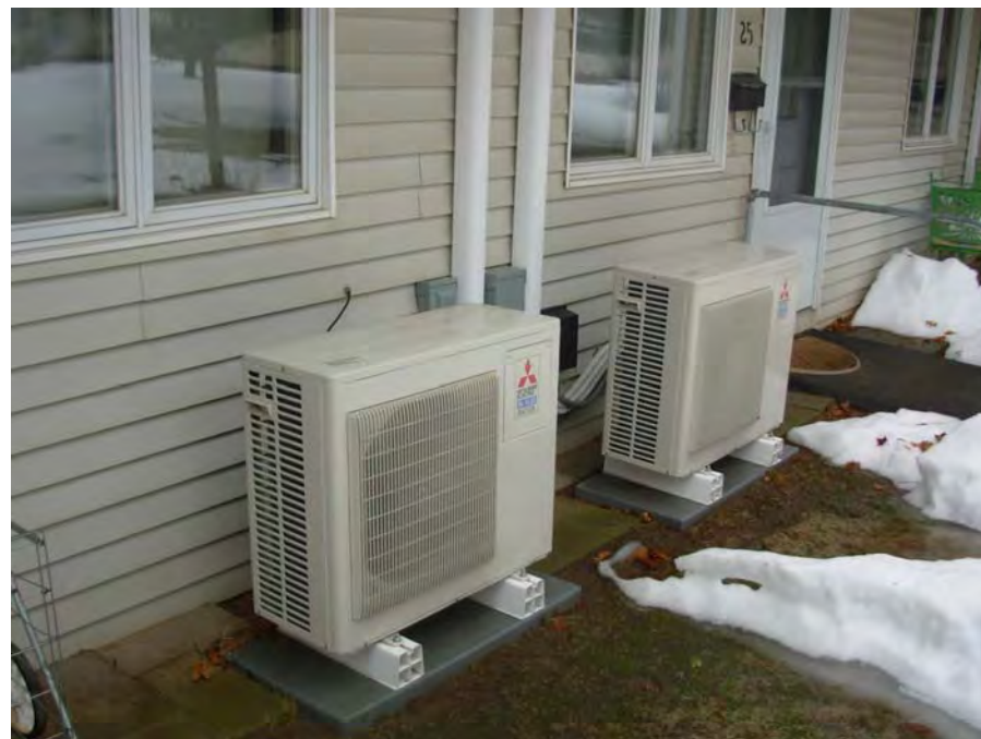
16. Typical heat pump HVAC system exterior condenser units
