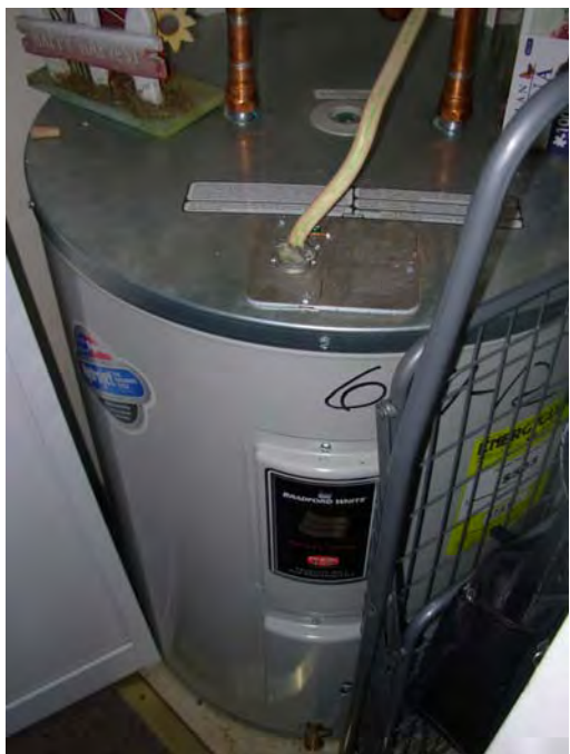
15. Typical DHW heater serving apartments
