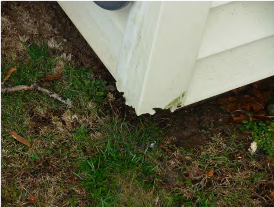
5. Most vinyl siding damage at grade level
